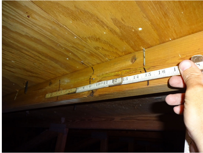
Figure 5 – Deck to Truss Attachment
