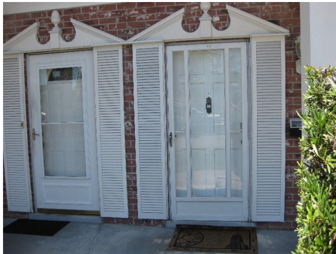
Figure 3 – Typical Front Door
