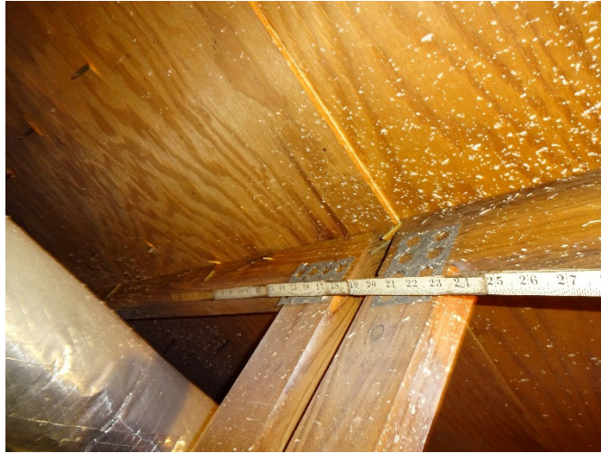
Figure 5 – Deck to Truss Attachment
