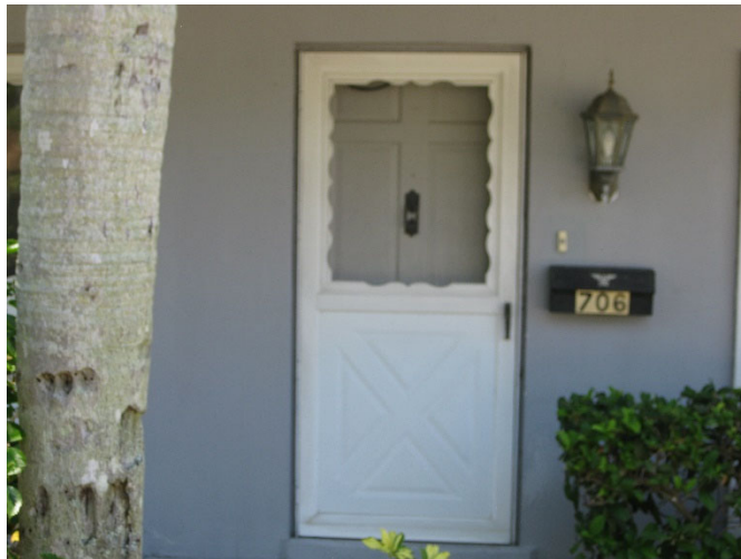
Figure 3 – Typical Front Door
