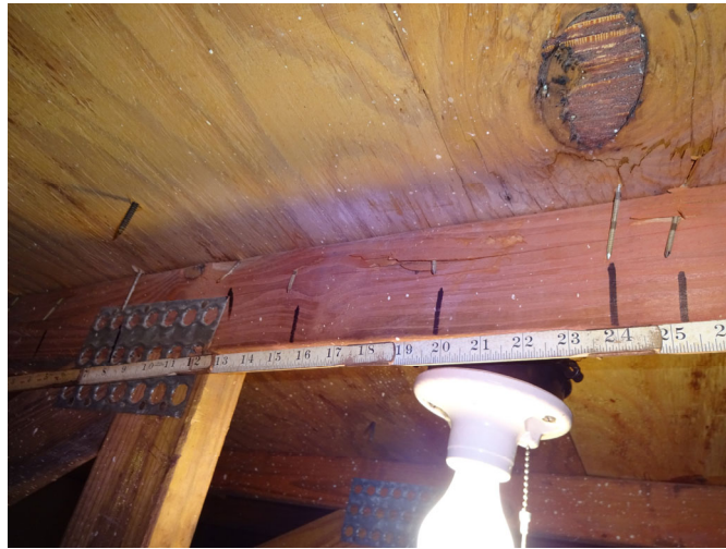
Figure 5 – Deck to Truss Attachment
