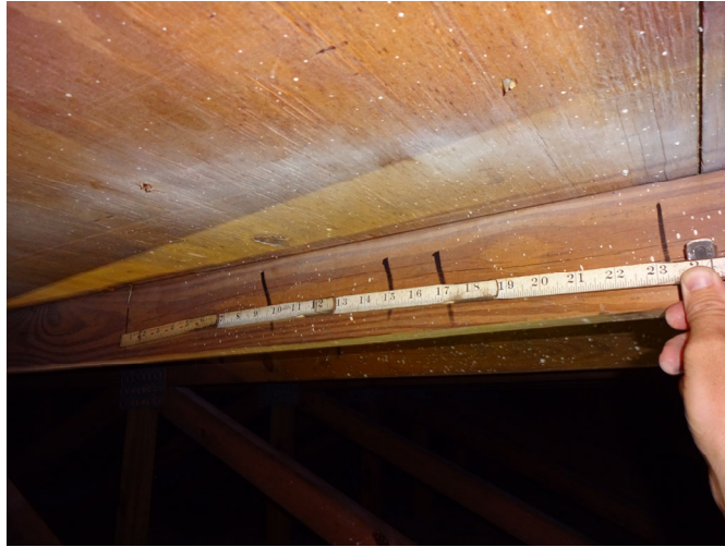
Figure 5 – Deck to Truss Attachment
