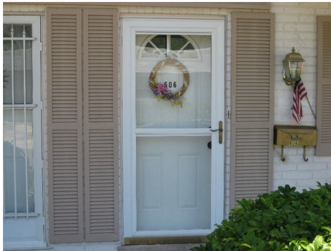
Figure 3 – Typical Front Door
