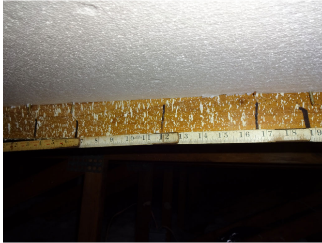
Figure 5 – Deck to Truss Attachment
