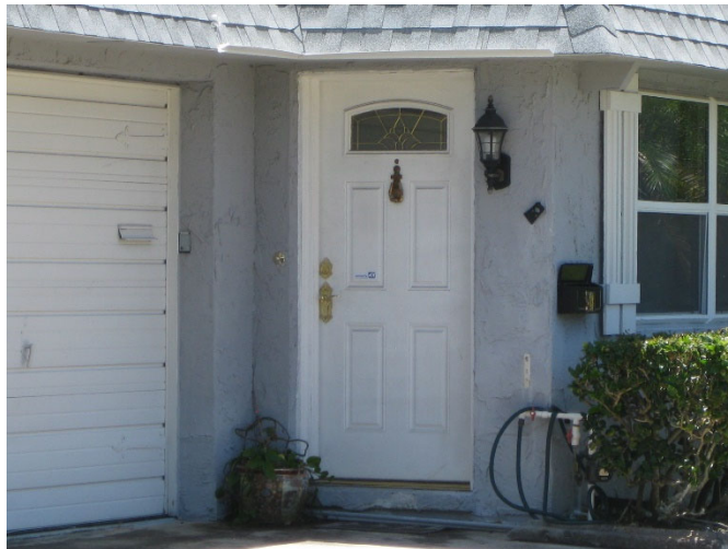
Figure 3 – Typical Front Door
