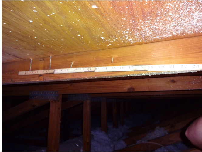
Figure 5 – Deck to Truss Attachment
