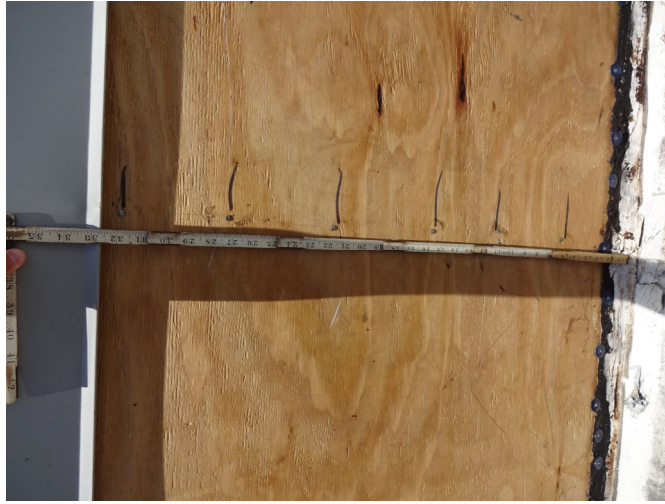
Figure 5- Deck to Truss Attachment
