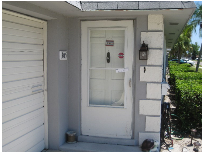
Figure 3 – Typical Front Door
