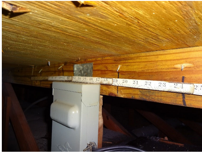
Figure 5 – Deck to Truss Attachment
