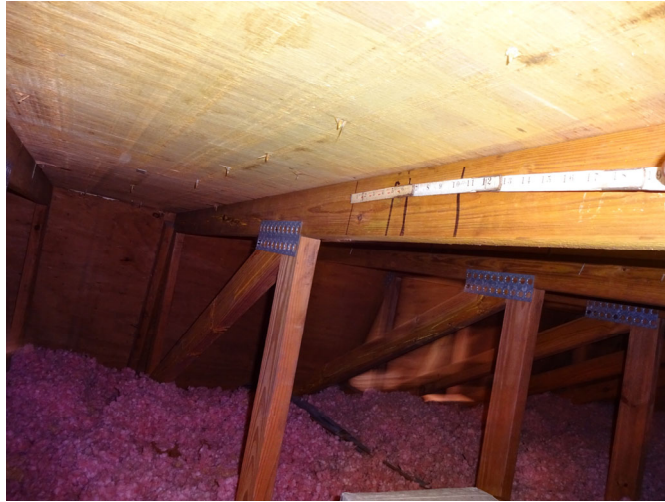
Figure 5 – Deck to Truss Attachment
