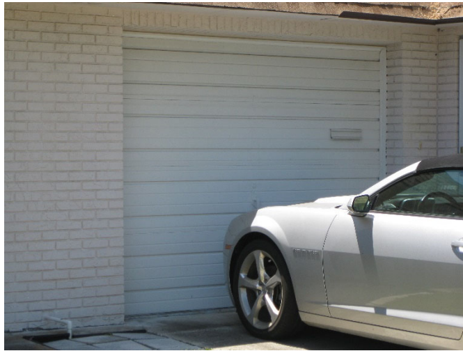
Figure 2 – Typical Garage Door
