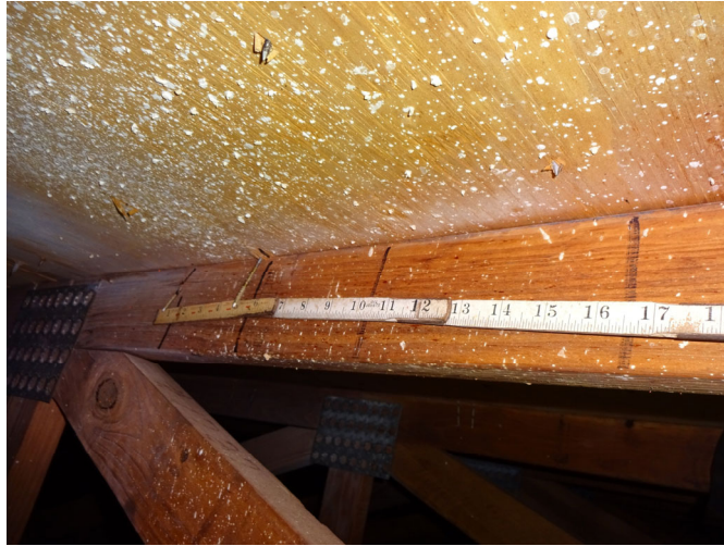
Figure 5 – Deck to Truss Attachment
