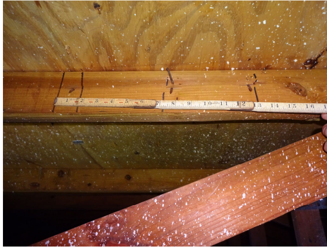
Figure 5 – Deck to Truss Attachment
