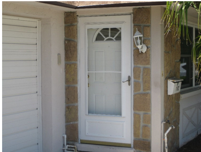
Figure 3 – Typical Front Door
