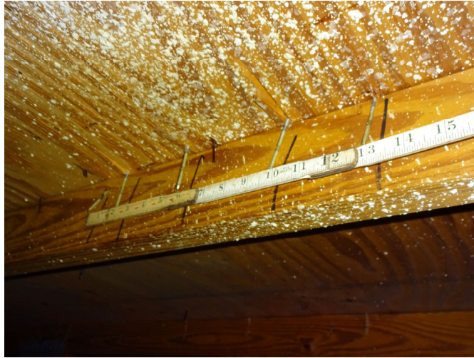
Figure 5 – Deck to Truss Attachment
