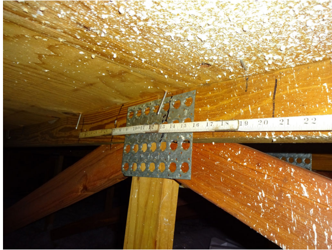
Figure 5 – Deck to Truss Attachment
