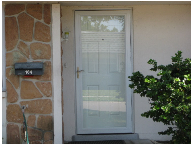
Figure 3 – Typical Front Door
