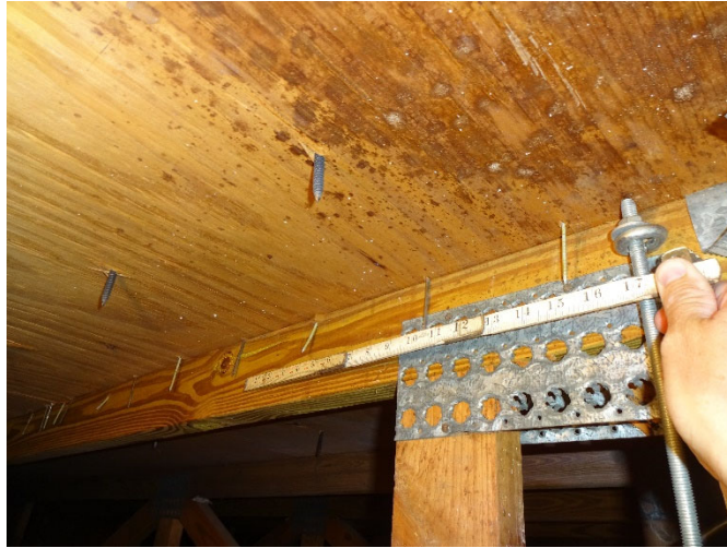
Figure 5 – Deck to Truss Attachment
